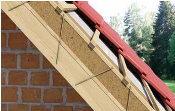
Fixing of soft over-rafter insulation
