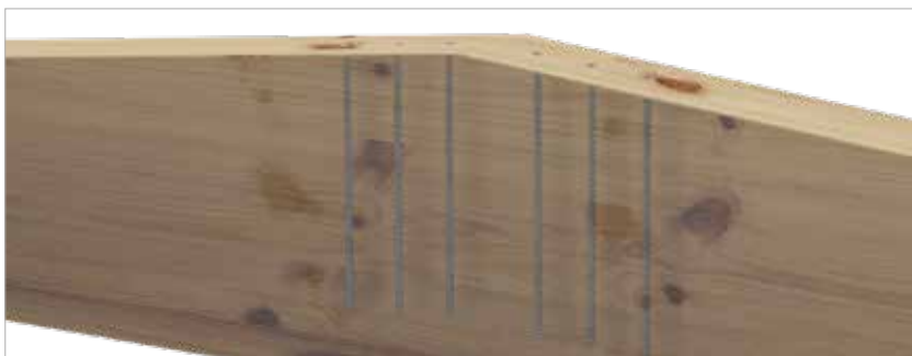
Reinforcement with screws in roof ridge area
