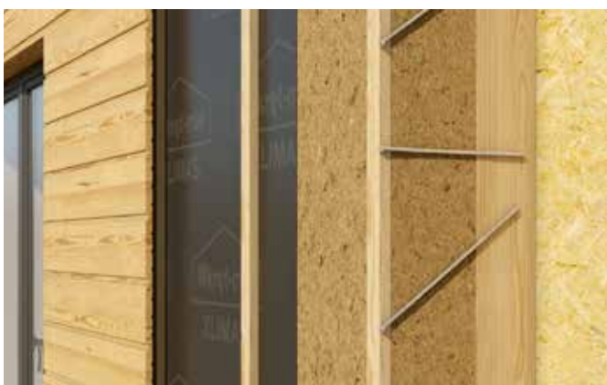
Fixing of insulation on façade
