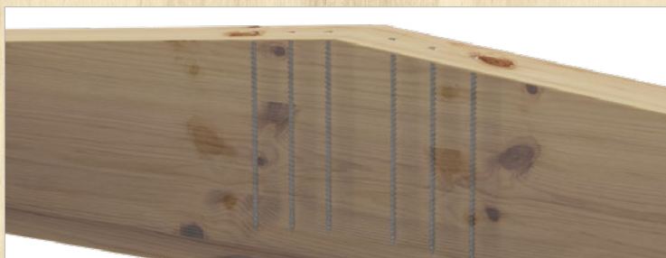
Reinforcement with screws in roof ridge area
